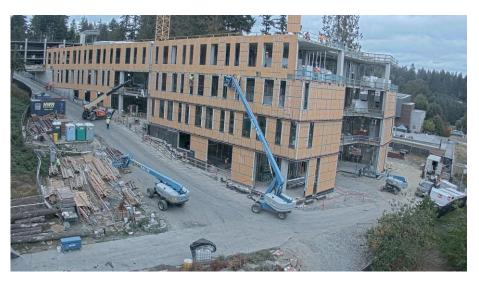
The roofing vapor barrier is complete which acts as a temporary roof during construction. The heavy mechanical screen framing has been delivered to site scheduled for erection last week of September.
