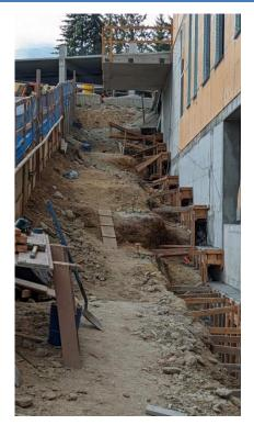
Concrete Corbels have been placed around the perimeter of the building for the masonry to bare on. Brick work is scheduled to start towards the end of next month. Also show above and below is the West Entrance balcony, which will provide a view point down the hill and into campus.
