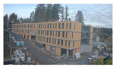
You may also notice from the above photo that the tower crane has been dismantled and removed. This is a big milestone for the project allowing the continuation of the building enclosure. The first two window water tests have been completed and passed with flying colors.
