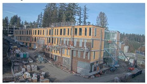
Masonry brick ledger is nearing completion. 75% of the brick ledger is fully welded off and inspected, to support the continuation of the brick façade. Below you can see brick installation in the southeast quadrant of the building.
