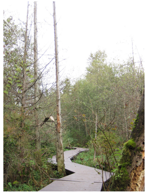
^ Here a dead western redcedar snag was left behind that should've been removed. While some curves in the route can be interesting, this part of the route would be better without so many of them.
