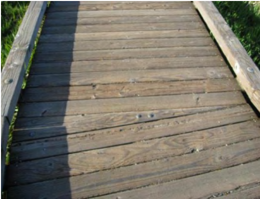
Photo 6.23: New boardwalk and flotation devices (Hanson 2012)
