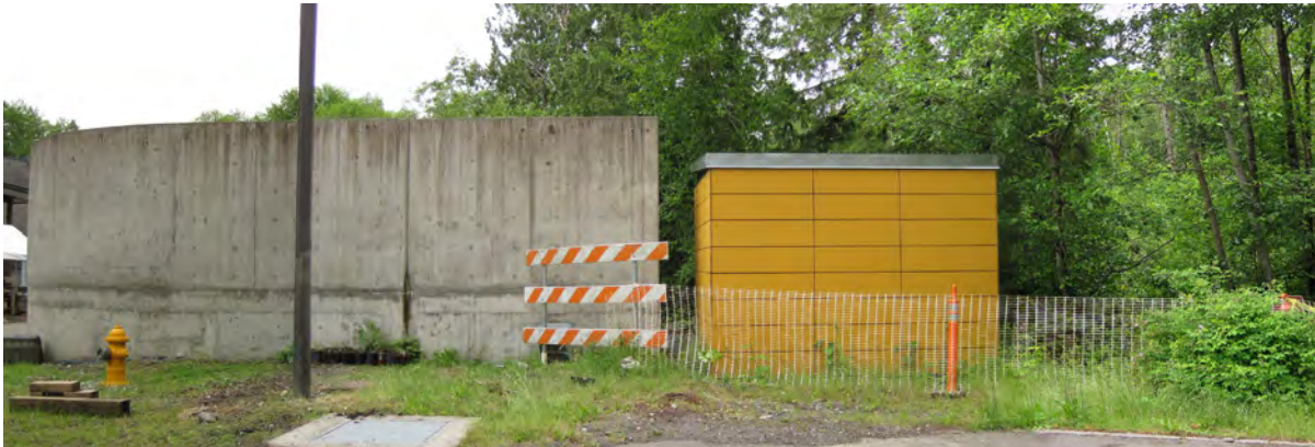
Figure 9.6: The main entry site's current condition (Hanson 2012)
