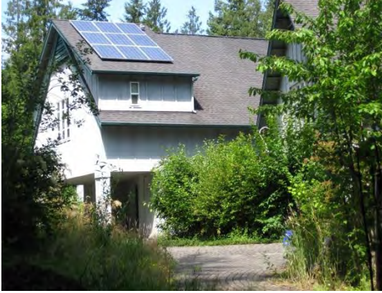
Photo 2.3: Northwest Stream Center (Hanson 2011)
