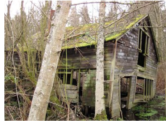
Photo 6.8: An interesting historic remnant building (Hanson 2012)
